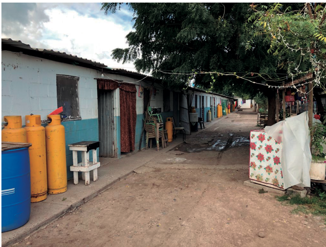
Photograph 1. Workers' Housing at a Large Grower's Headquarters
