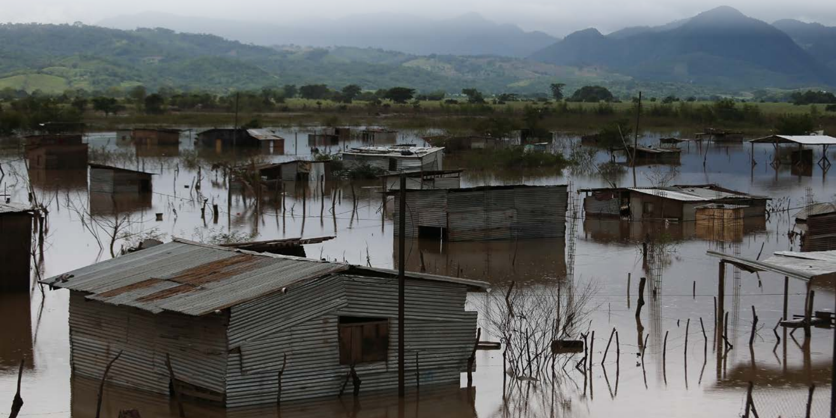
While moving inland, Hurricane ETA weakened into a tropical storm, but the unrelenting and heavy rains it carried caused extensive floods, landslides, and massive damages in Nicaragua, Guatemala, Honduras, and Panama. Image source: EU, 2020 (D. Membreño) / Flickr (CC BY-NC 2.0)
