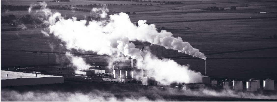
ROCHELLE, ILLINOIS, AUGUST 2010: The Illinois River Energy biofuels plant in Rochelle releases plumes of steam at sunrise. The ethanol plant processes over 40 million bushels of corn into 115 million gallons of fuel grade ethanol annually. The plant is one of hundreds around the country transforming corn into ethanol. It takes nearly 1,000 gallons of water to produce a gallon of ethanol from irrigated corn: four gallons from unirrigated corn. Photo © J. Carl Ganter / Circle of Blue
